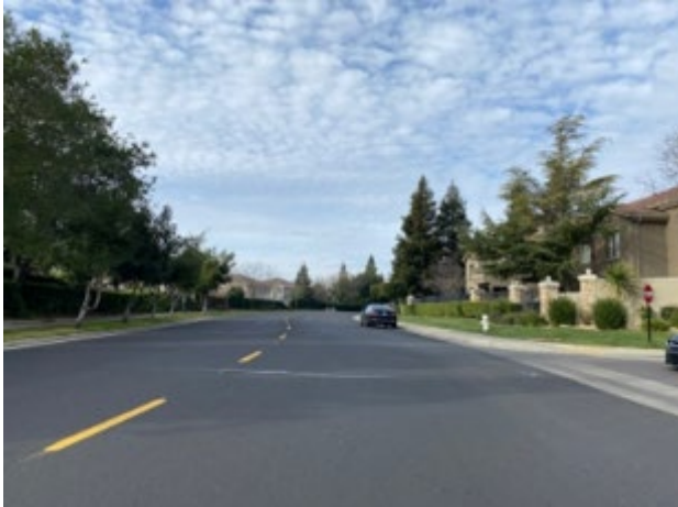
View north on East Taron Road
