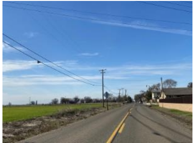
View west on Poppy Ridge Road
