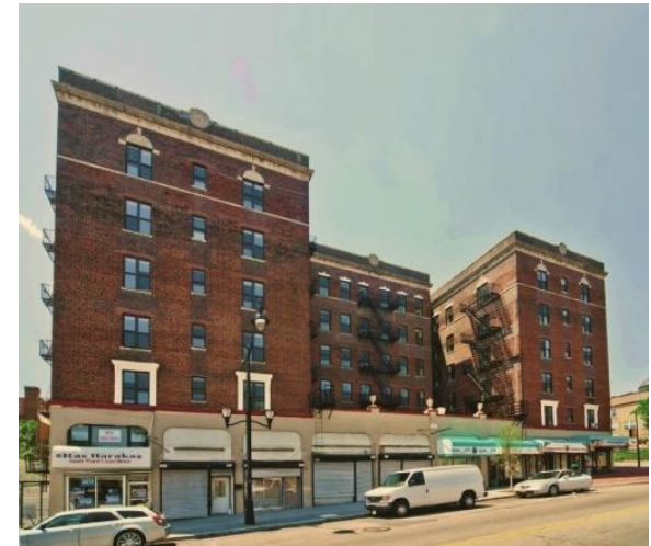
2 Osborne Terrace Newark, NJ
